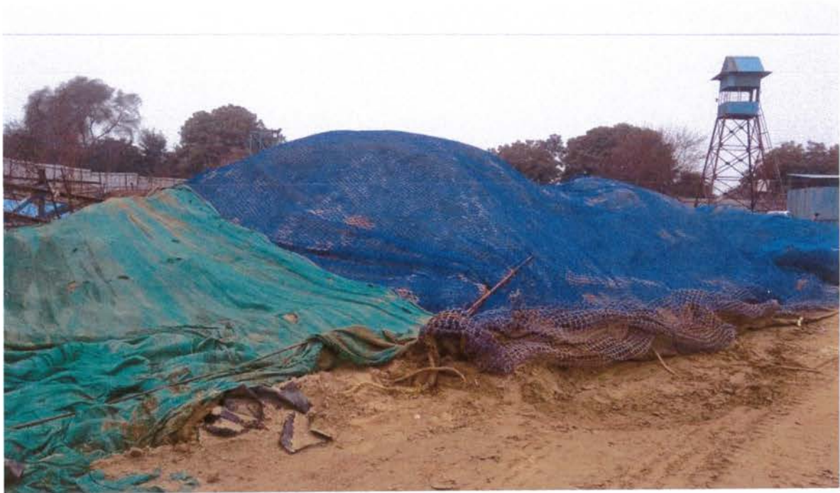
2.3 covered loose soil heap at ESS
