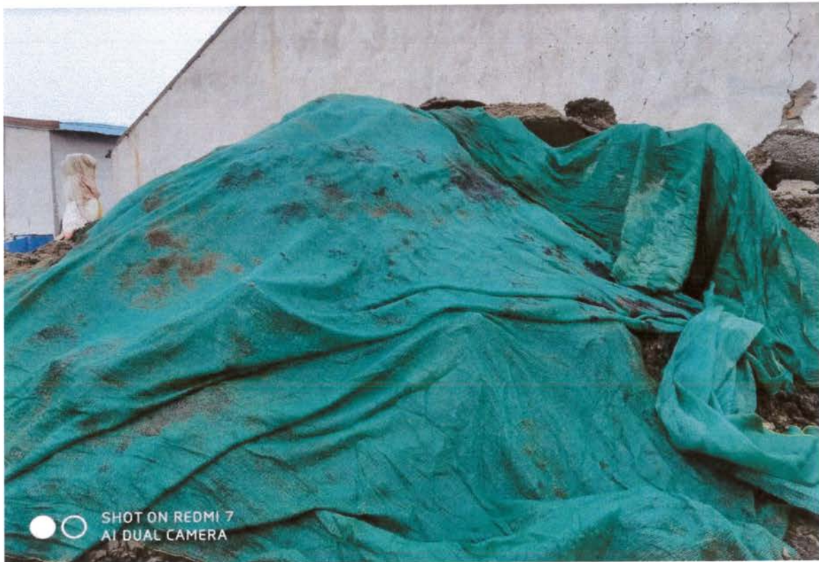
1.2 construction and demolition waste dumped at designated place and covered
