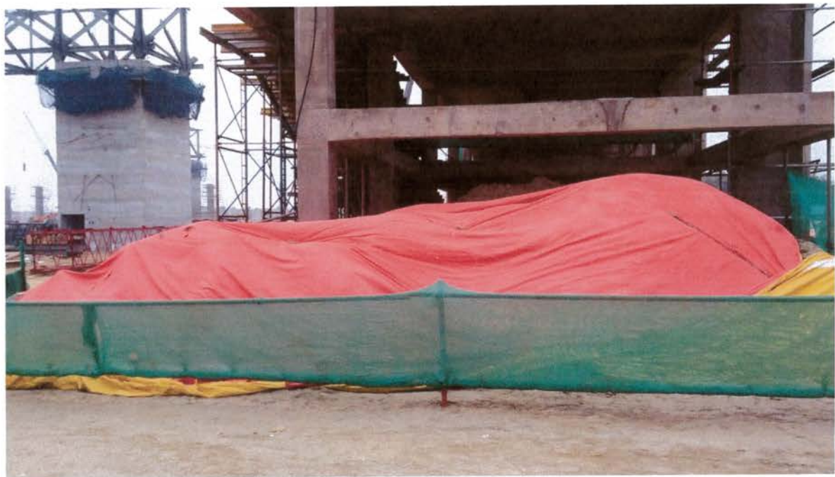
2.1 Covered aggregate at batching plant
