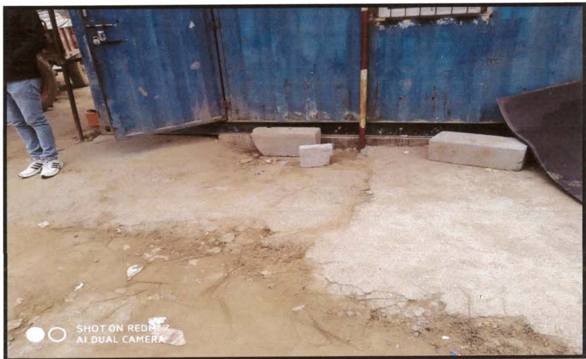
1.3. Use of construction and demolition waste in developing pavement near site offices
