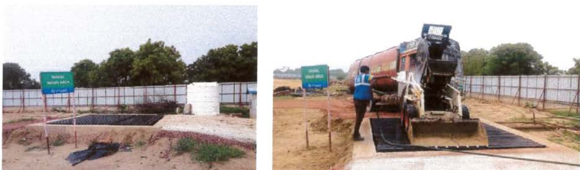
Figure 10B: Wheel-wash area to clean construction vehicles' dust/mud-laden tyres
