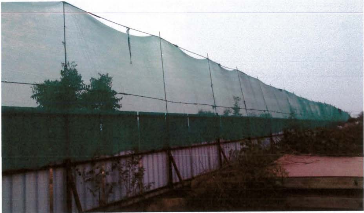
5. increased barricading height
