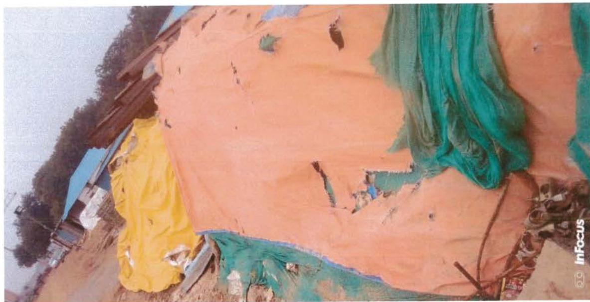
2.4 Covered loose material at time office
