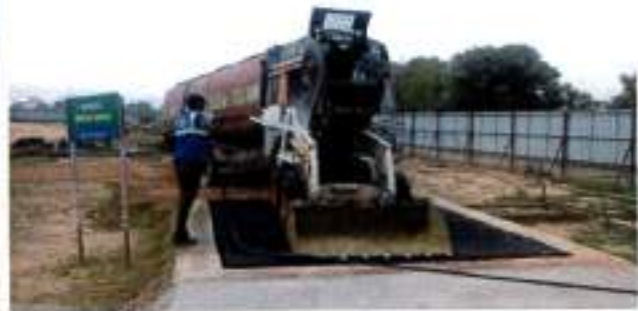
Figure 10B: Wheel wash area to clean construction vehicles' wheels
