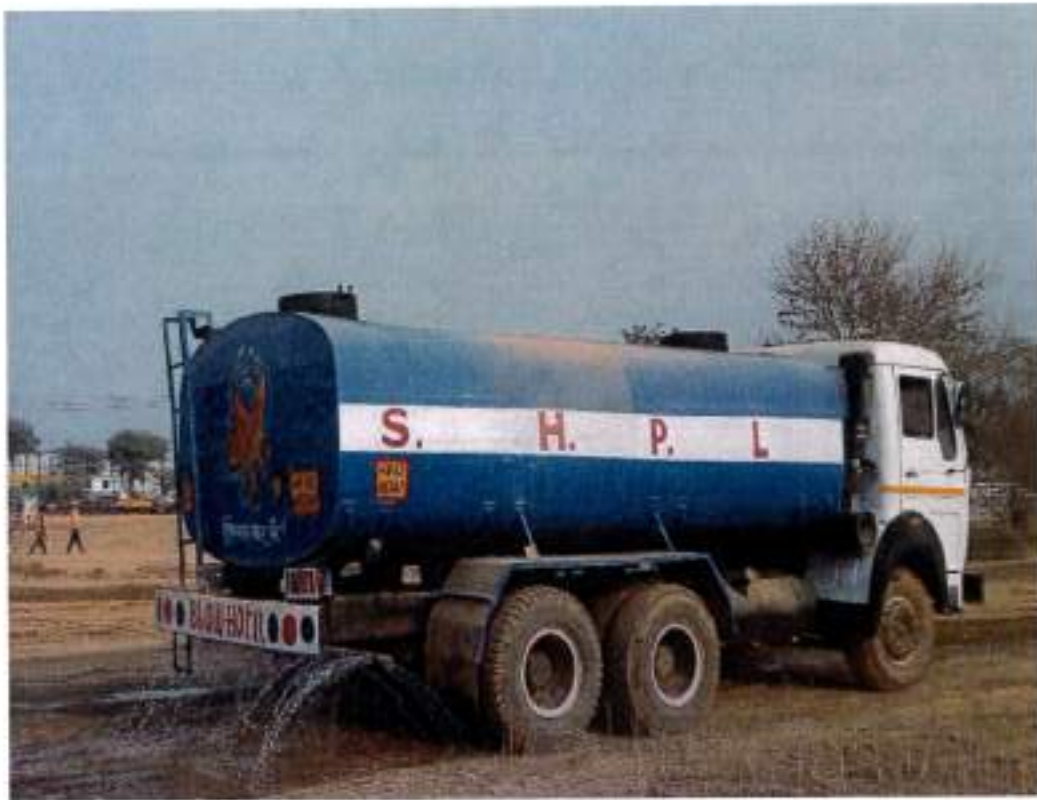
Figure 10A: Dust Suppression through sprinkling of water
