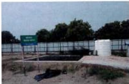
Figure 10B: Wheel wash area to clean construction vehicles' wheels
