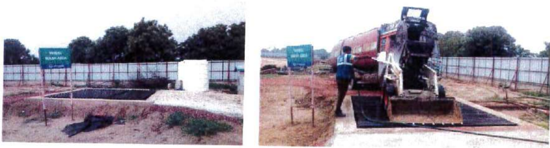
Figure 10B: Wheel-wash area to clean construction vehicles' dust/mud-laden tyres
