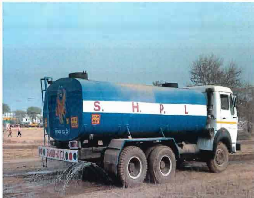
Figure 10A: Dust Suppression through sprinkling of water
