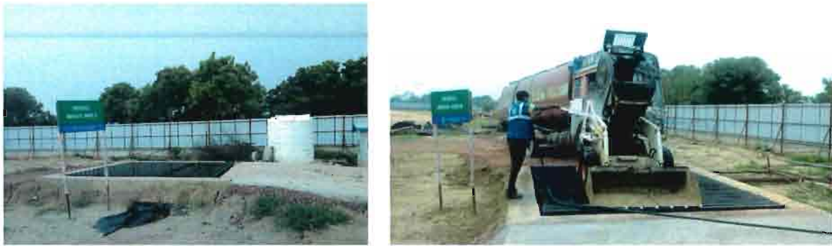
Figure 10B: Wheel-wash area to clean construction vehicles' dust/mud-laden tyres
