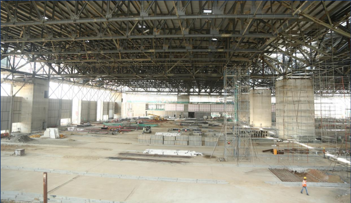
Exhibition Hall 01- PHE Trench & Grade Slab in Progress
